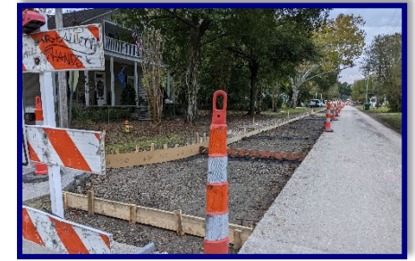
Carey Street Pavement Reconstruction
